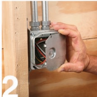
2 Step 2: Hook feet on right side or bottom of plate
